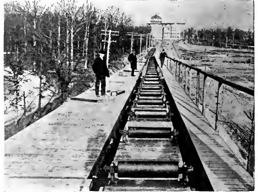
FIG. 1.—CARRIERS USED IN TWO-BELT CONVEYOR.
